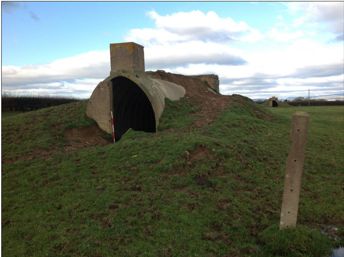
Plate 107: The rear of shelter PRN 04447s, with the unknown concrete post in the foreground.
