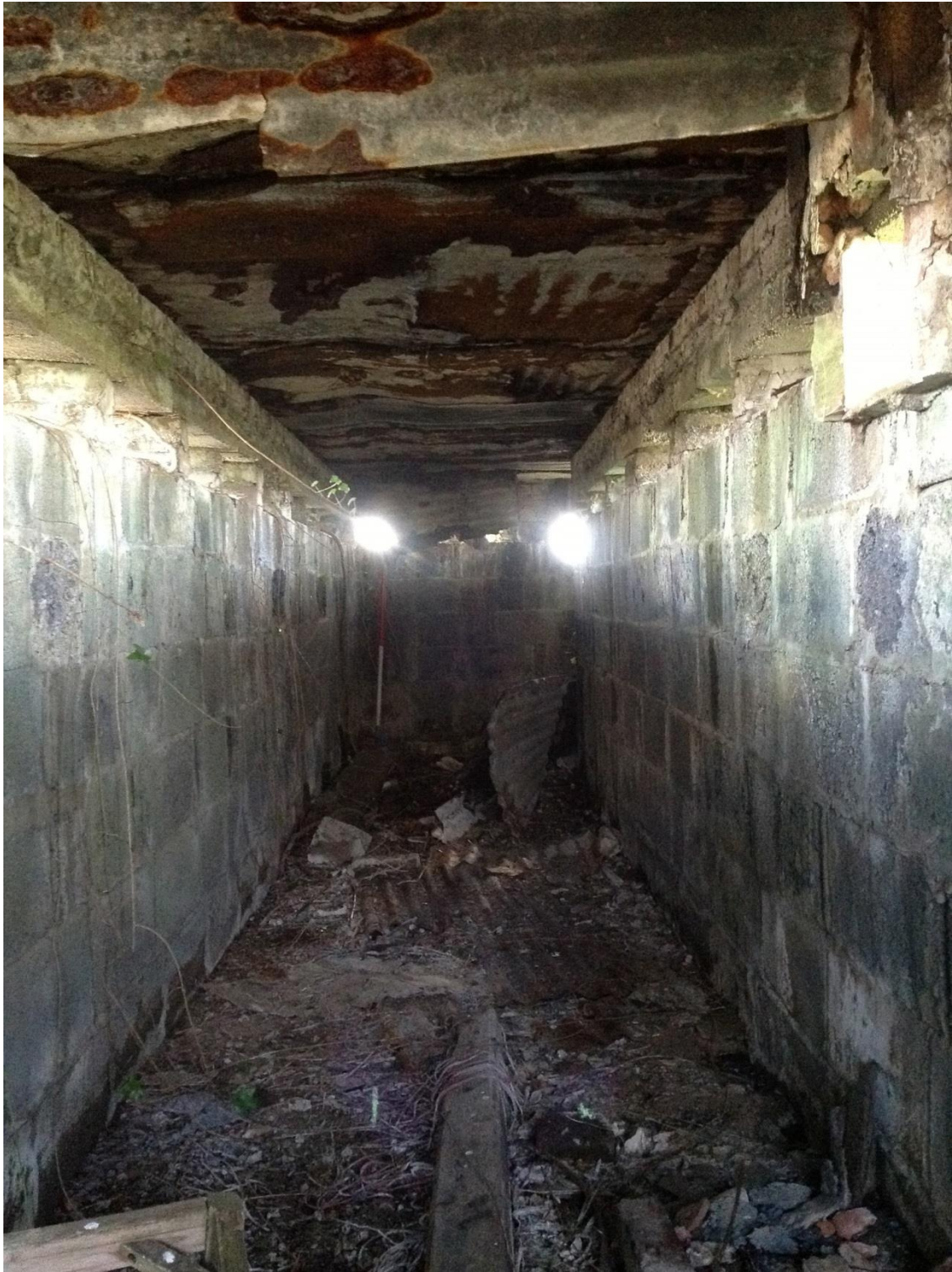
Plate 66: Interior of PRN 07395m. Note the blockwork construction.
