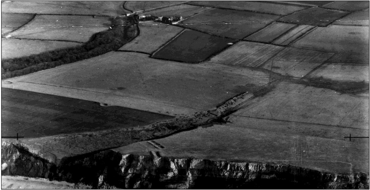
Plate 85: Anti-landing obstacles set out in fields to the south of the Landing Ground.
