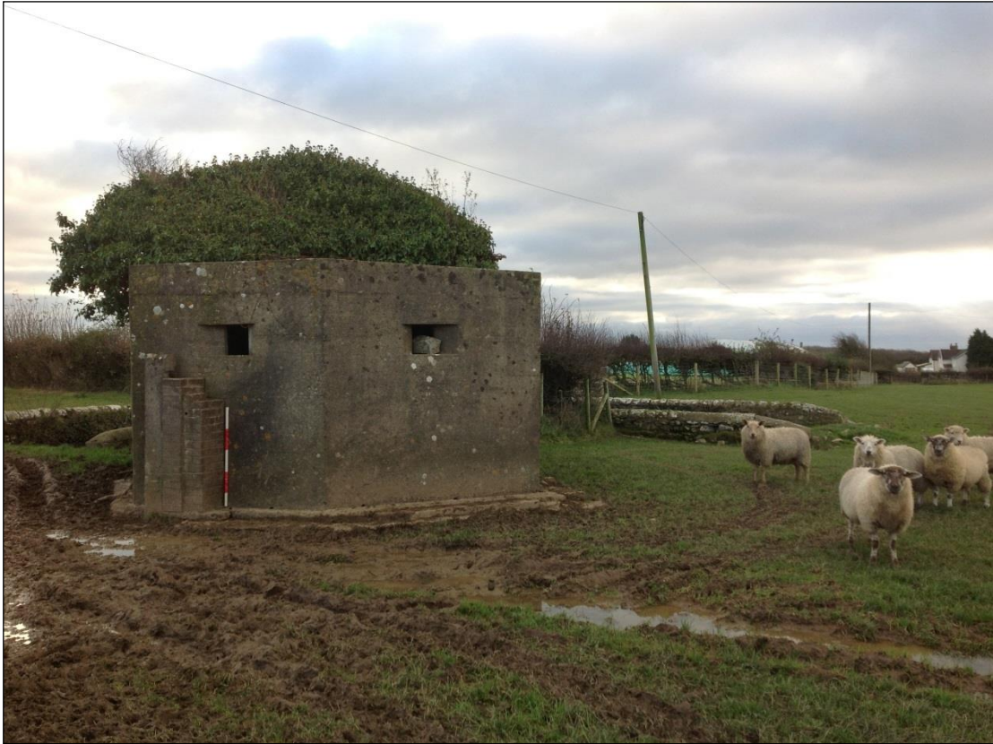
Plate 132: The north facing elevation of pillbox 04468s. Note the concrete and brick dais on which the structure stands.
