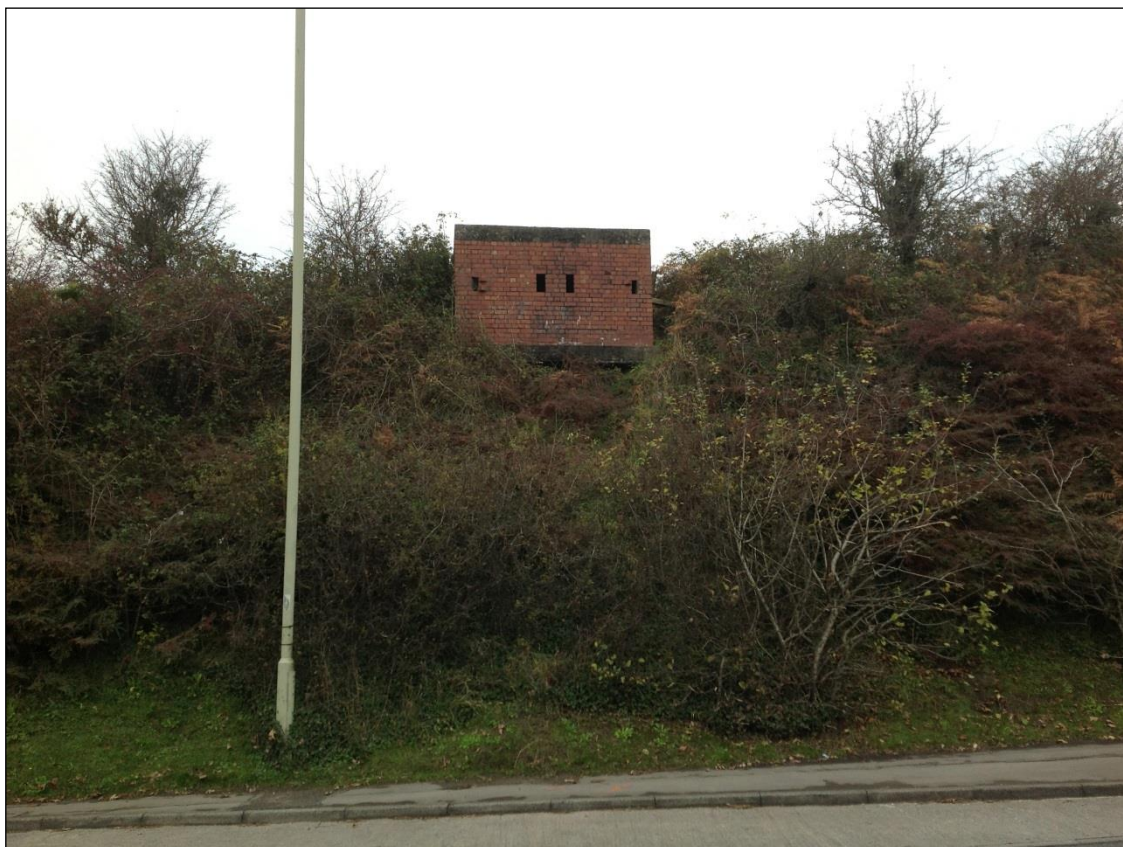
Plate 58: The southeast facing elevation of PRN 07390m.
