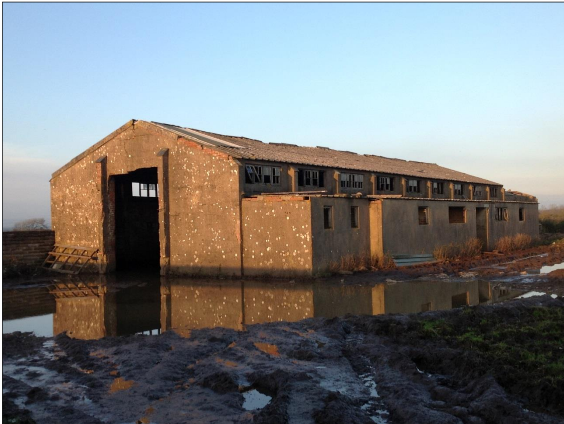
Plate 89: Gymnasium and Chapel building. View to the north.
