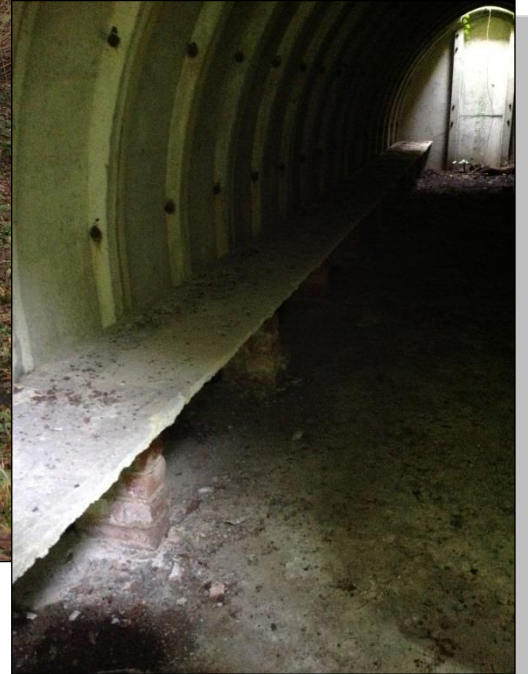
Plate 10: Air raid shelter. Concrete skimmed internal seating.
