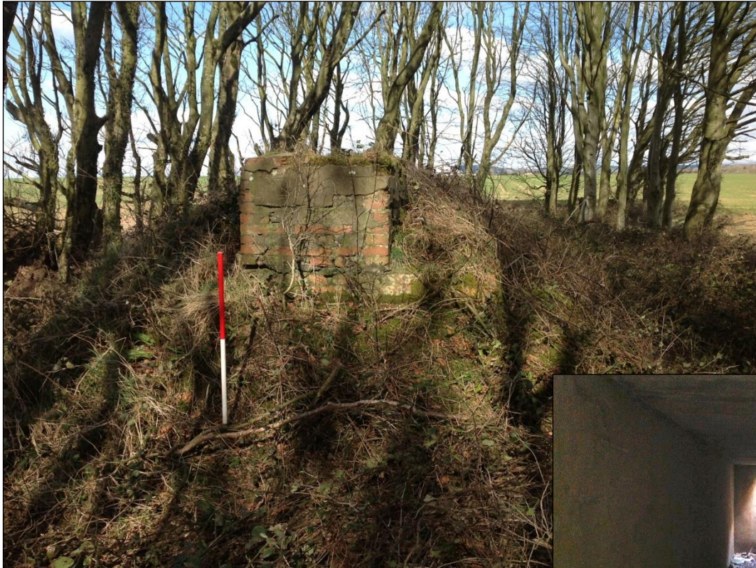
Plate 72: (Above) The brick escape hatch at the southern end of the munitions store. (Right) The Interior of the store. Note the 'C' ring style rungs at the rear of the structure.
