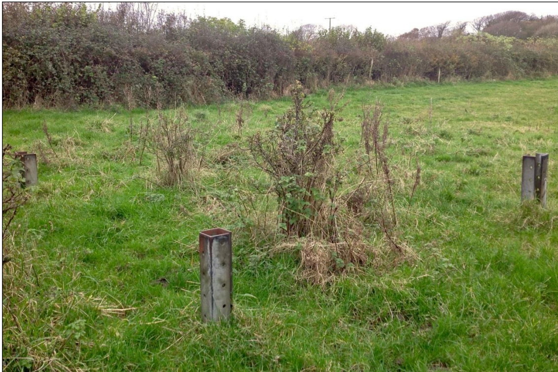
Plate 130: Remains of the posts that anchored one of the VHF aerials
