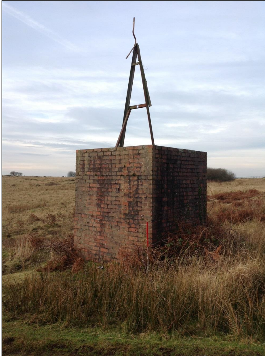
Plate 50: The southern airfield beacon PRN 06770w.
