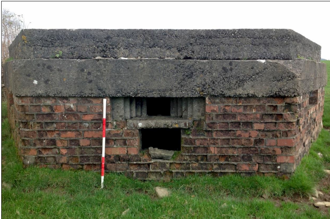
Plate 135: The west facing loopholes. The top is for fitted with a Turnbull mount for Vickers MG, while the lower is for 'Boys' anti-tank rifle.
