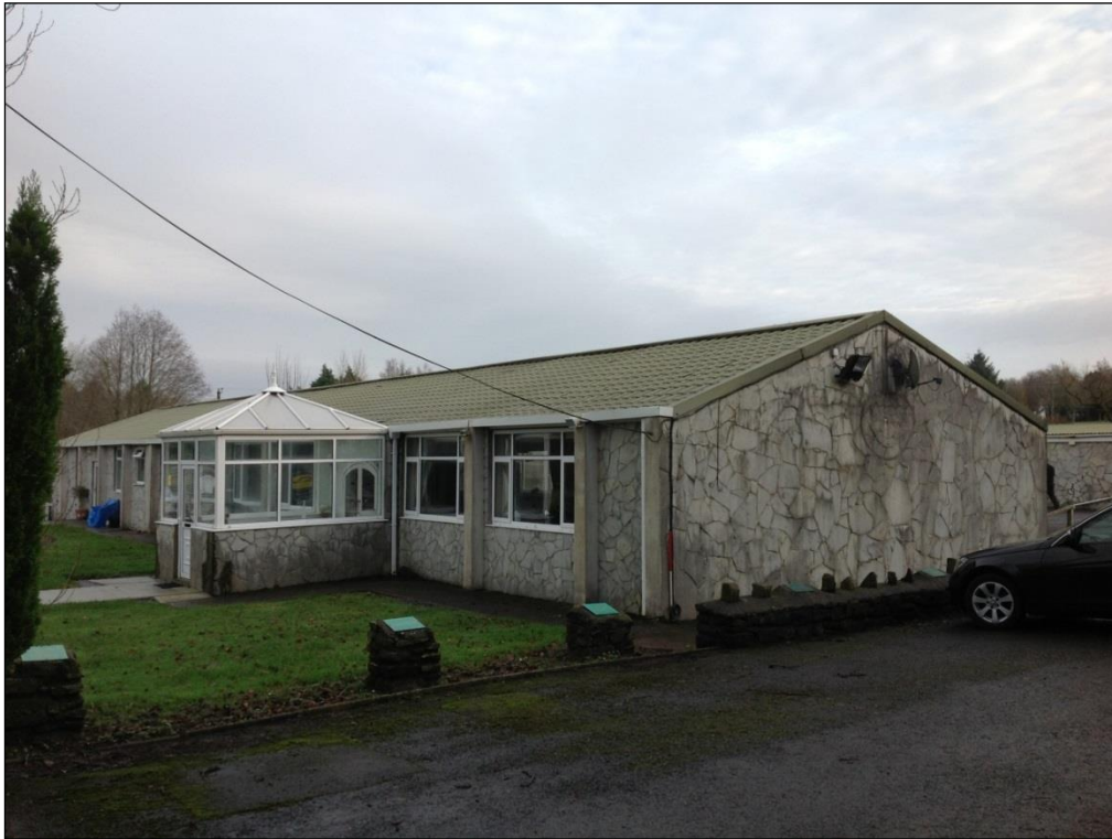
Plate 17: The Ward block building which forms the western half of the Sick Quarters.
