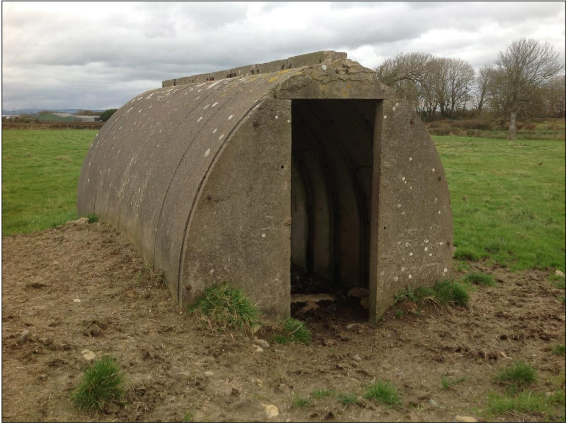
Plate 115: The main entrance to the air raid shelter PRN 04455s.
