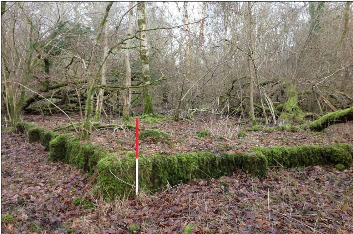
Plate 152: Remains of the concrete plinth for the Crew Room. View to the northwest.
