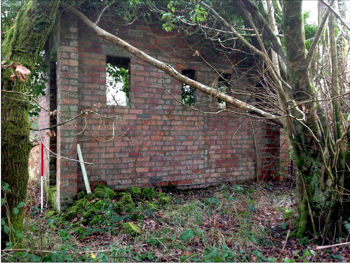
Plate 13: The range of four windows along the frontal elevation of the latrine block.
