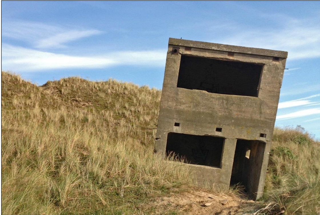
Plate 78: The remaining quadrant tower of the Margam training range: Not the angle of the building
