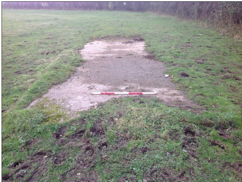
Plate 105: The concrete base of building 59.
