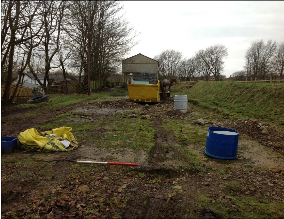
Plate 36: A heavily damaged concrete apron is all that survives of PRN 07843w.
