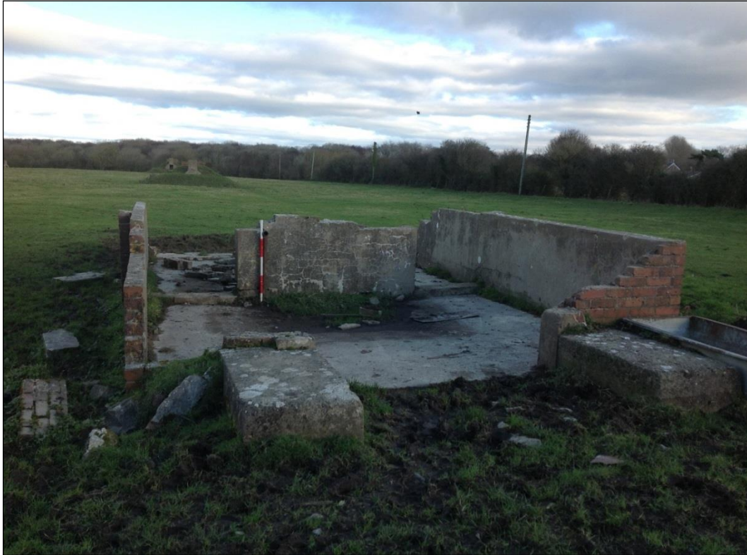
Plate 95: The remains of the sites bucket emptying platform.
