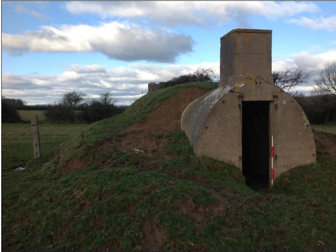
Plate 102: Rear of the air raid shelter PRN 04442s. Note the concrete post associated with the structure on the left.
