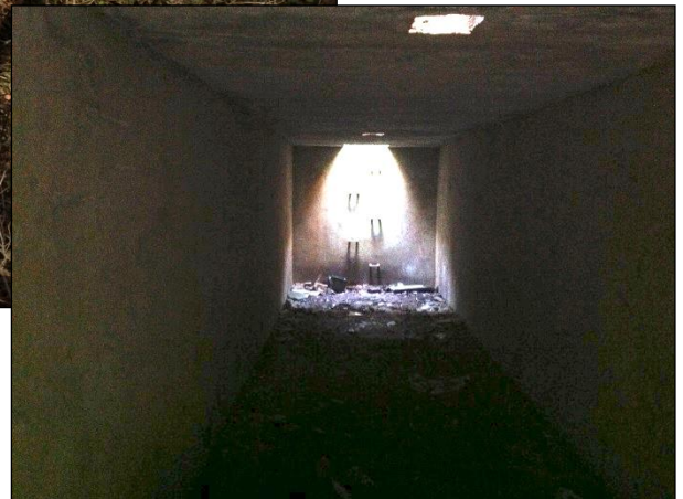
Plate 72: (Above) The brick escape hatch at the southern end of the munitions store. (Right) The Interior of the store. Note the 'C' ring style rungs at the rear of the structure.
