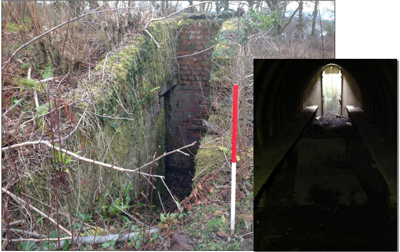
Plate 15: The second of the two Stanton shelters on the WAAF site.
