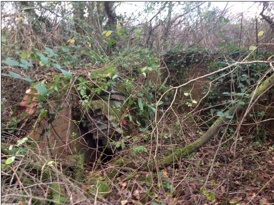
Plate 160: The northwest facing entrance to the blast shelter.
