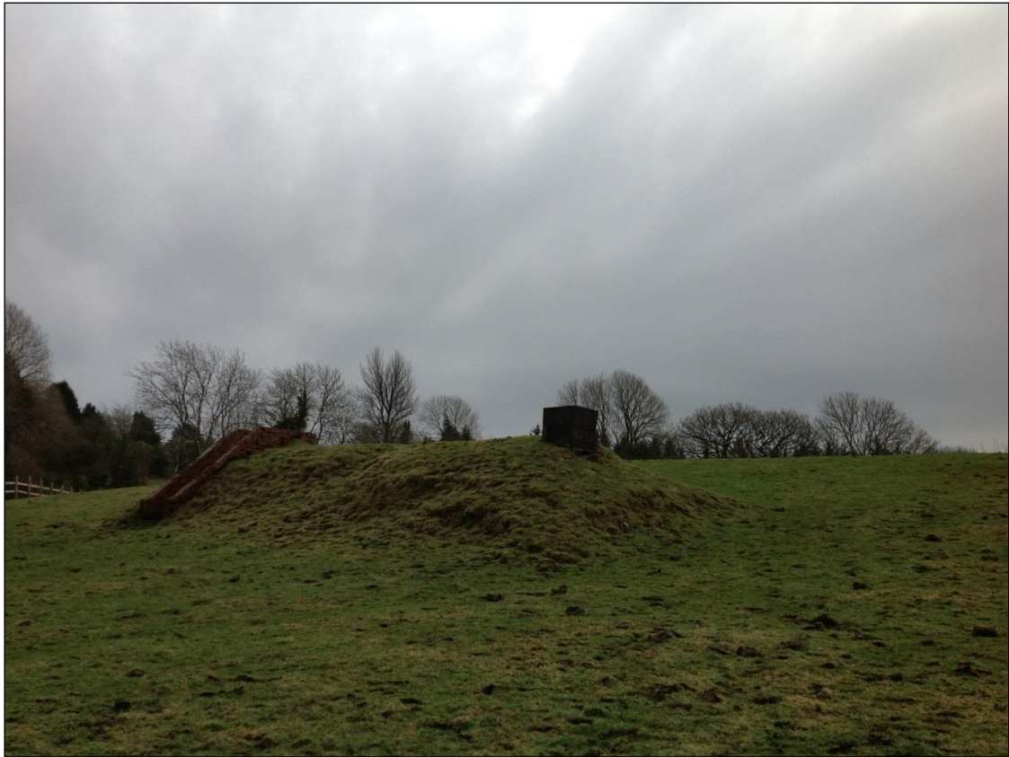
Plate 39: Stanton Air Raid Shelter. View to the east.
