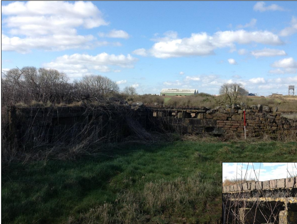
Plate 62: Loop-holed wall. (Inset) Detail of the embrasures.
