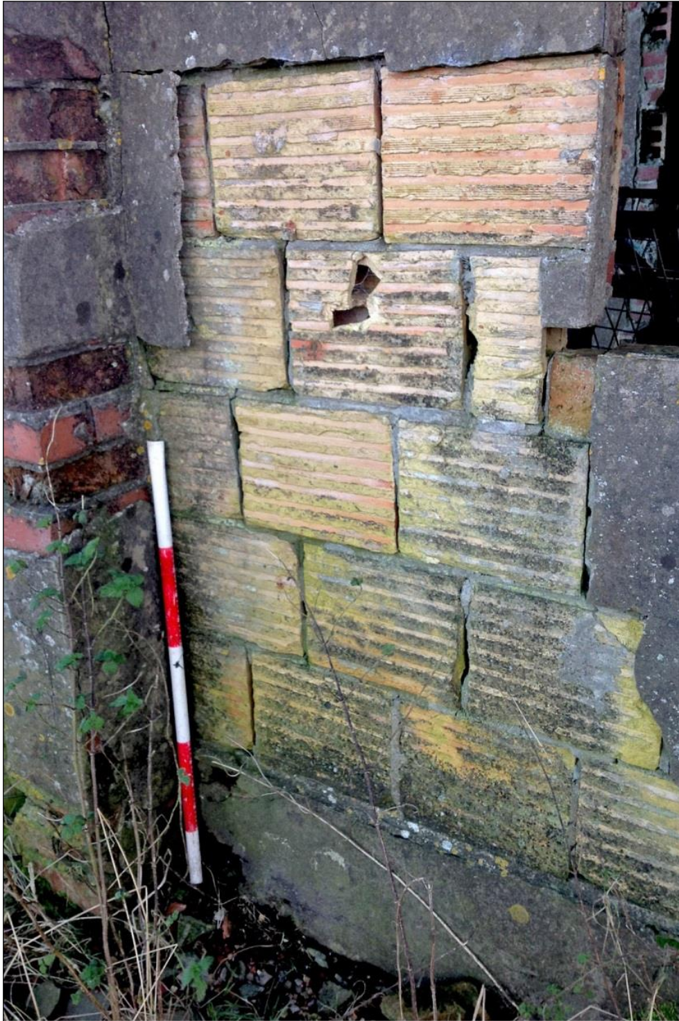
Plate 140: Detail of the eastern extension, showing the pale yellow hollow terra cotta blocks, usually employed for internal partitions.
