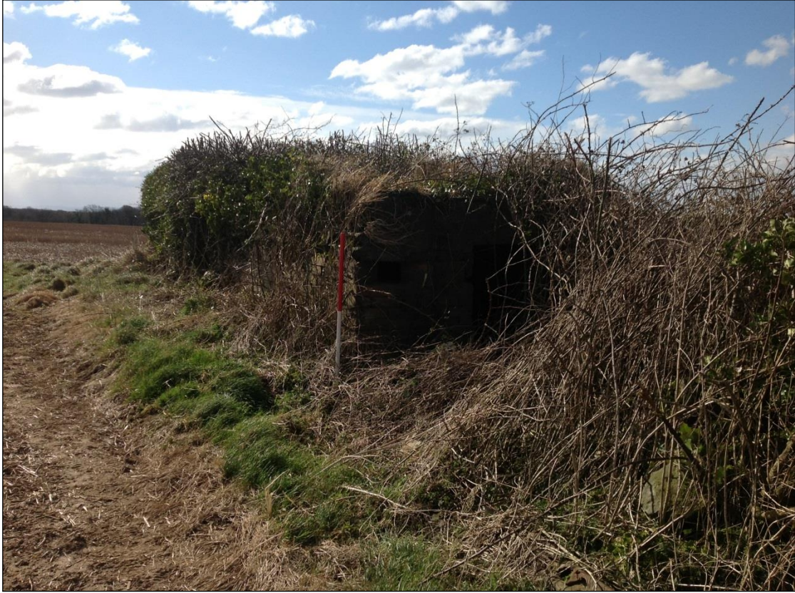
Plate 65: The entrance to the section trench. View to the south.
