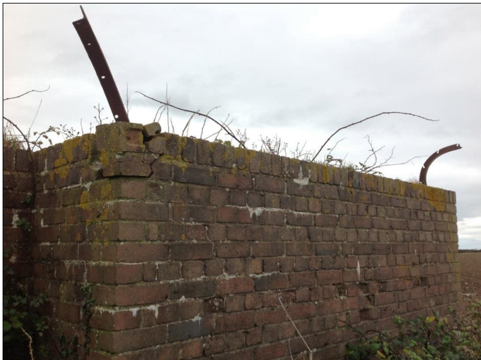
Plate 125: Cast iron posts extend from the top corners of the wall to act as a deterrent
