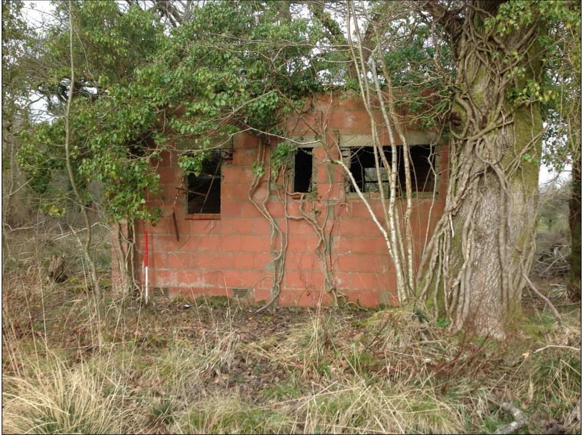
Plate 11: Front elevation of the sergeant's latrine block
