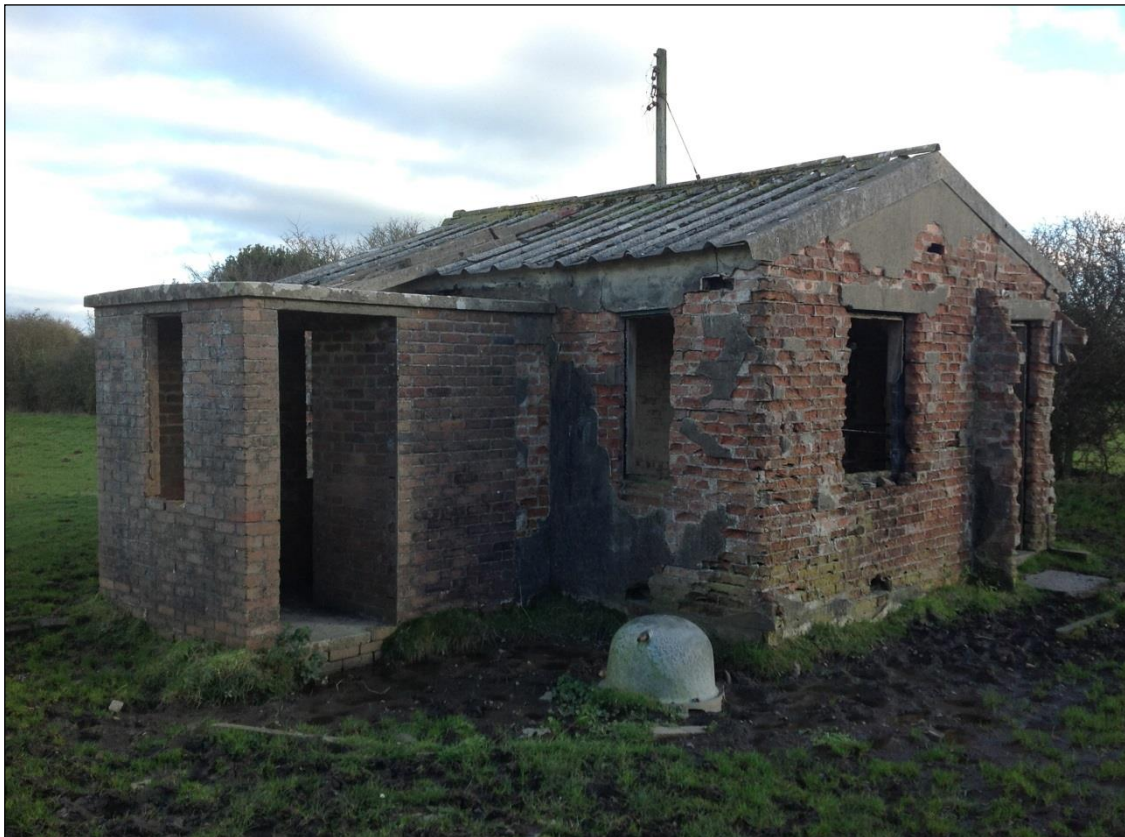
Plate 94: Picket Post (PRN 04434s). East facing elevation.
