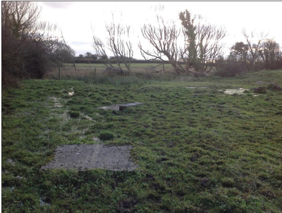
Plate 101:Disappearing fast: Very little remains of building 48 as it sinks beneath boggy ground.
