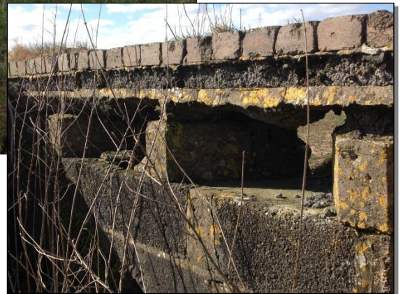
Plate 62: Loop-holed wall. (Inset) Detail of the embrasures.
