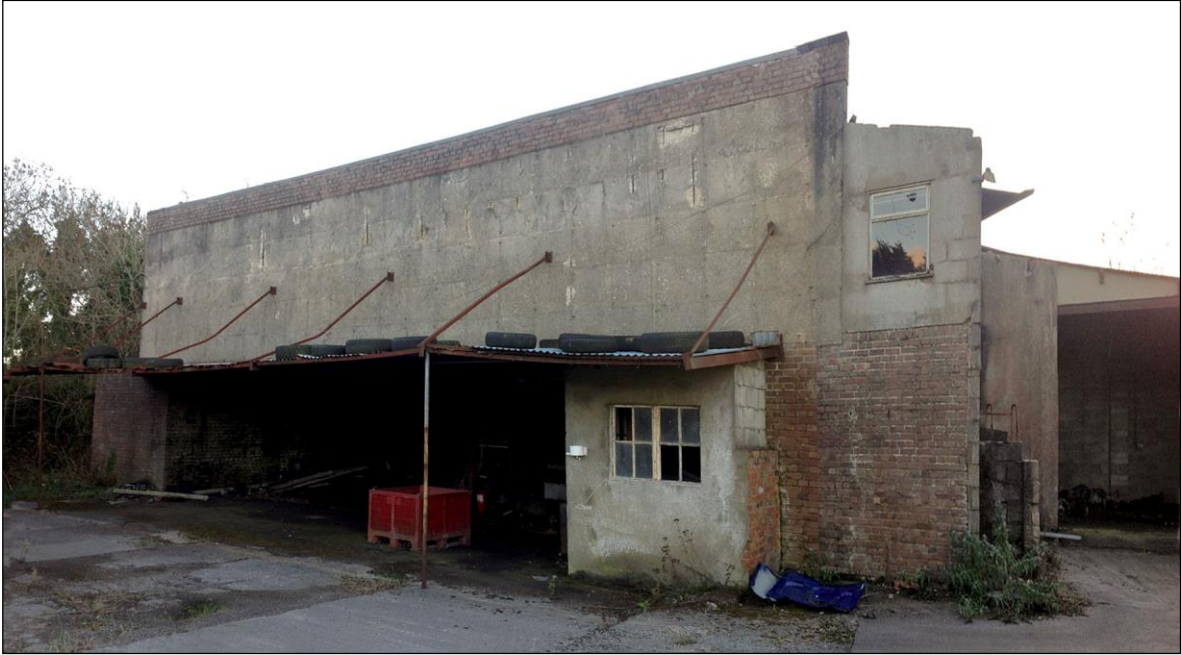
Plate 157: Northeast facing elevation of the Aircraft MG Test Butts.
