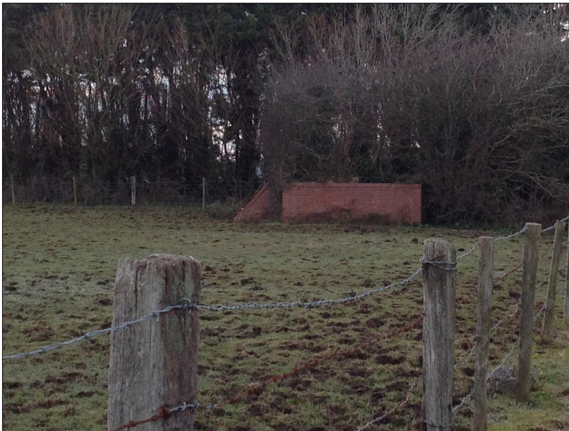
Plate 91: A brick blast shelter located towards the northeast boundary of Site No.1
