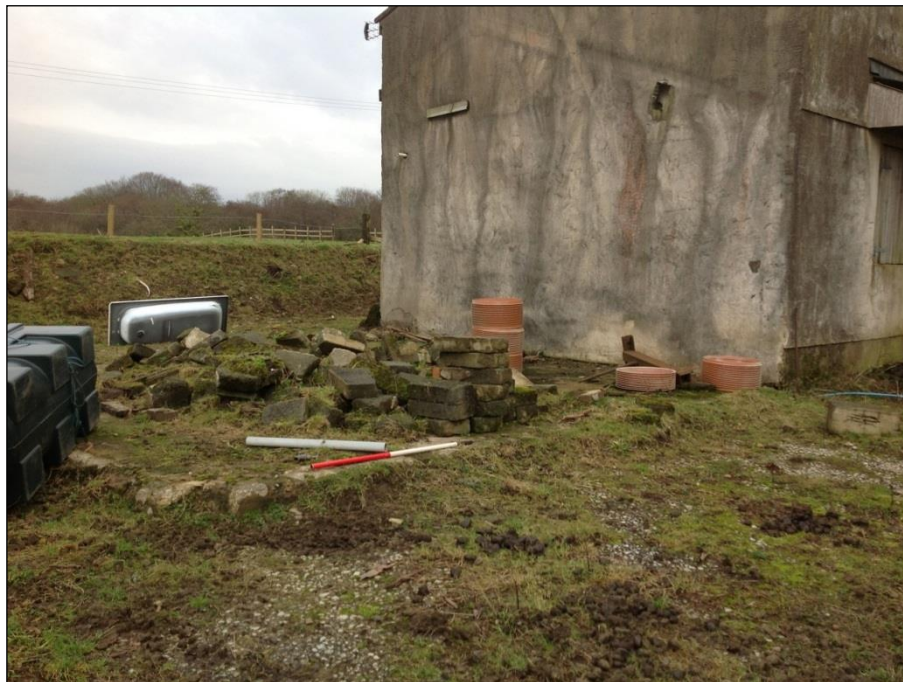
Plate 37: Little now remains of the building 151.
