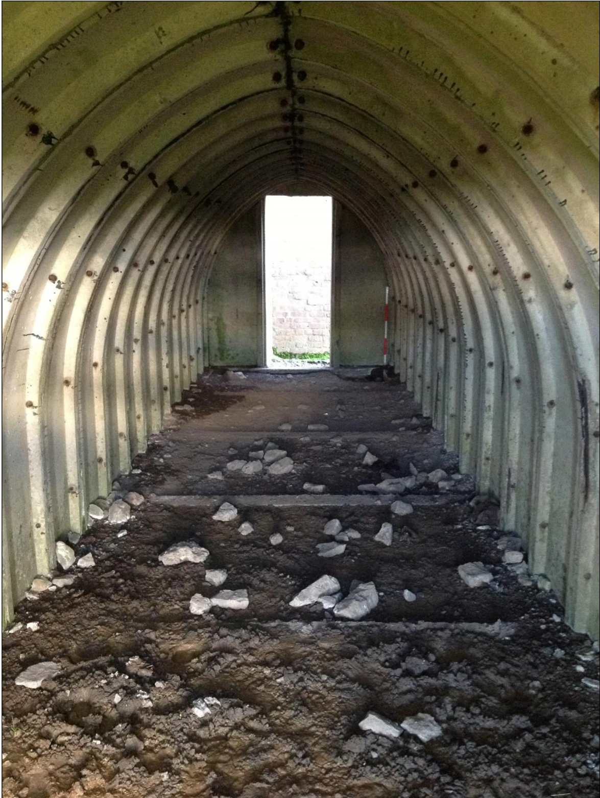
Plate 99: The interior of PRN 04439s. Note the pre-cast concrete sections which bolted together to form a tunnel of the required length.
