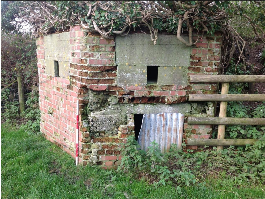
Plate 133: The east facing elevation of Pillbox 04469s.
