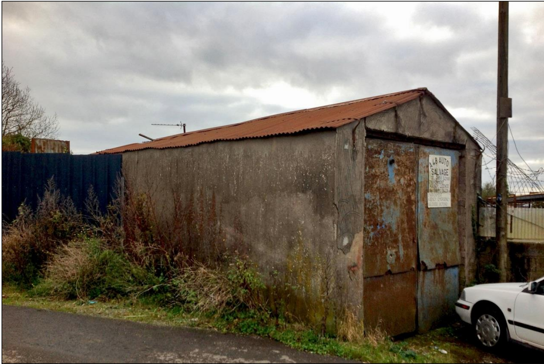
Plate 156: Building of unknown use. View to the west.
