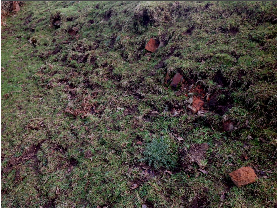
Plate 16: Demolition rubble is all that remains of the Operations Blocks water tank
