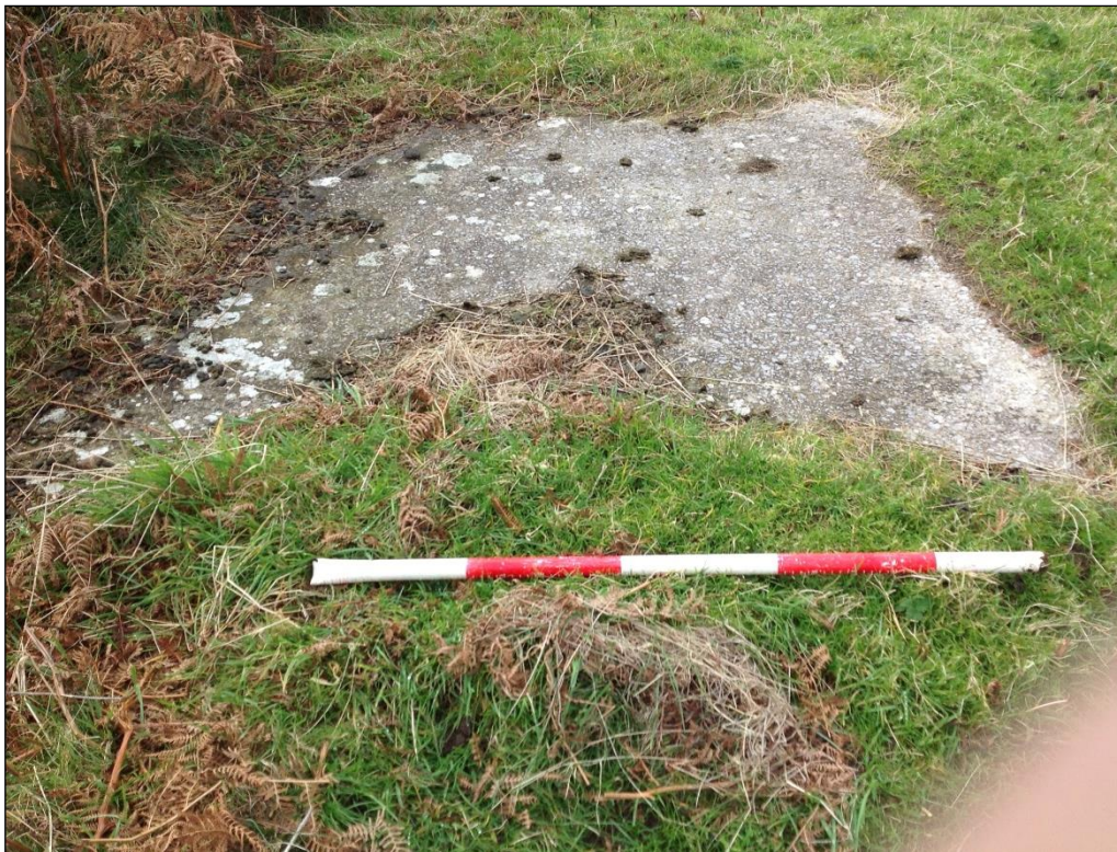
Plate 83: A small square concrete apron of unknown use.
