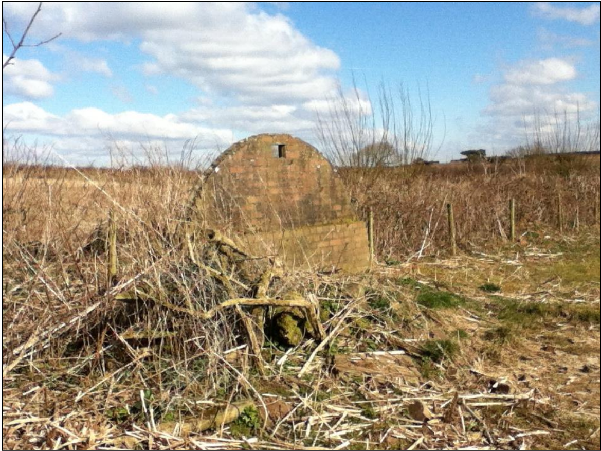
Plate 71: Remains of the rear end of a Turners curved asbestos hutting structure.
