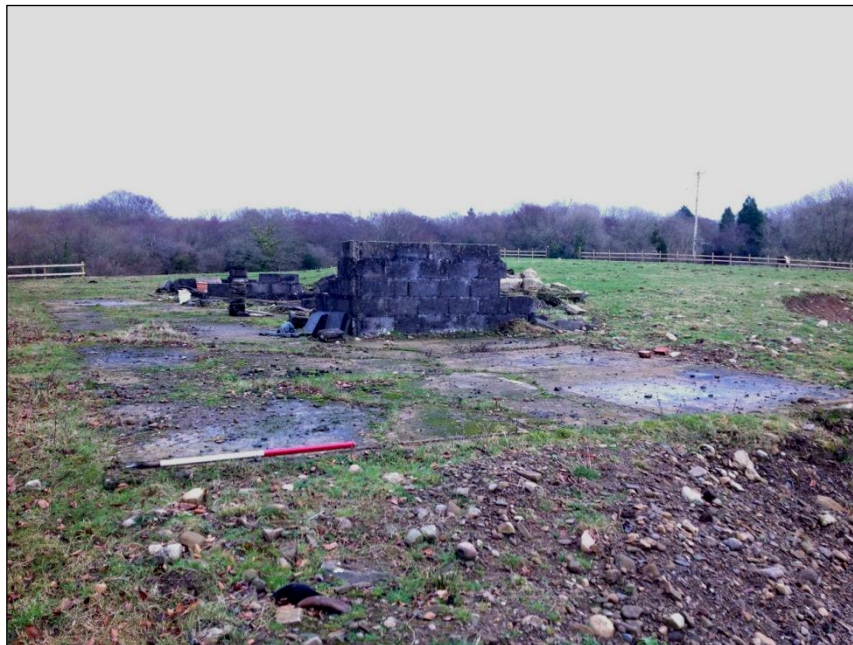
Plate 38: Heavily damaged airmens quarters. View to the north.
