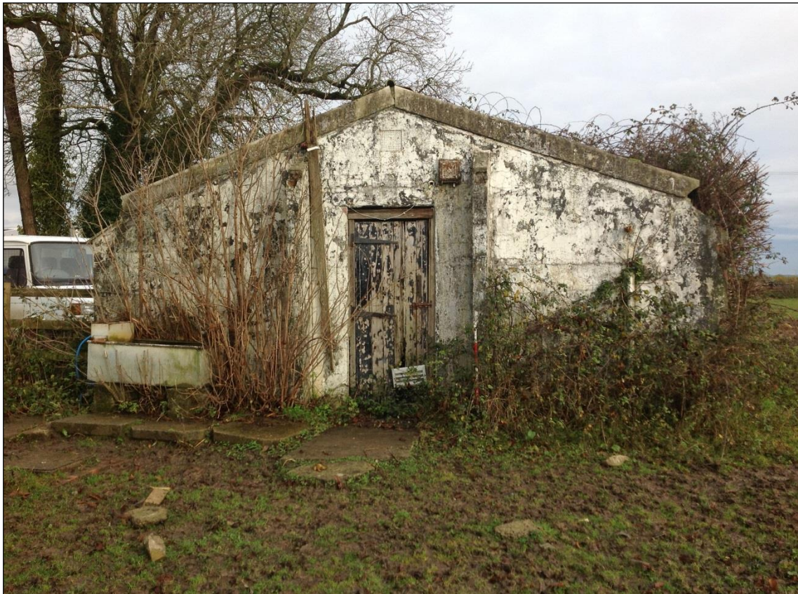
Plate 120: The southwest facing gable end of the Airwomen's Quarters building. Note the remains of buildings telegraph pole to the left of the doorway.
