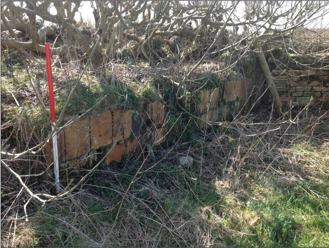
Plate 69: Hollow terra cotta blocks (usually employed for internal partitions) have been used to construct this defensive feature.
