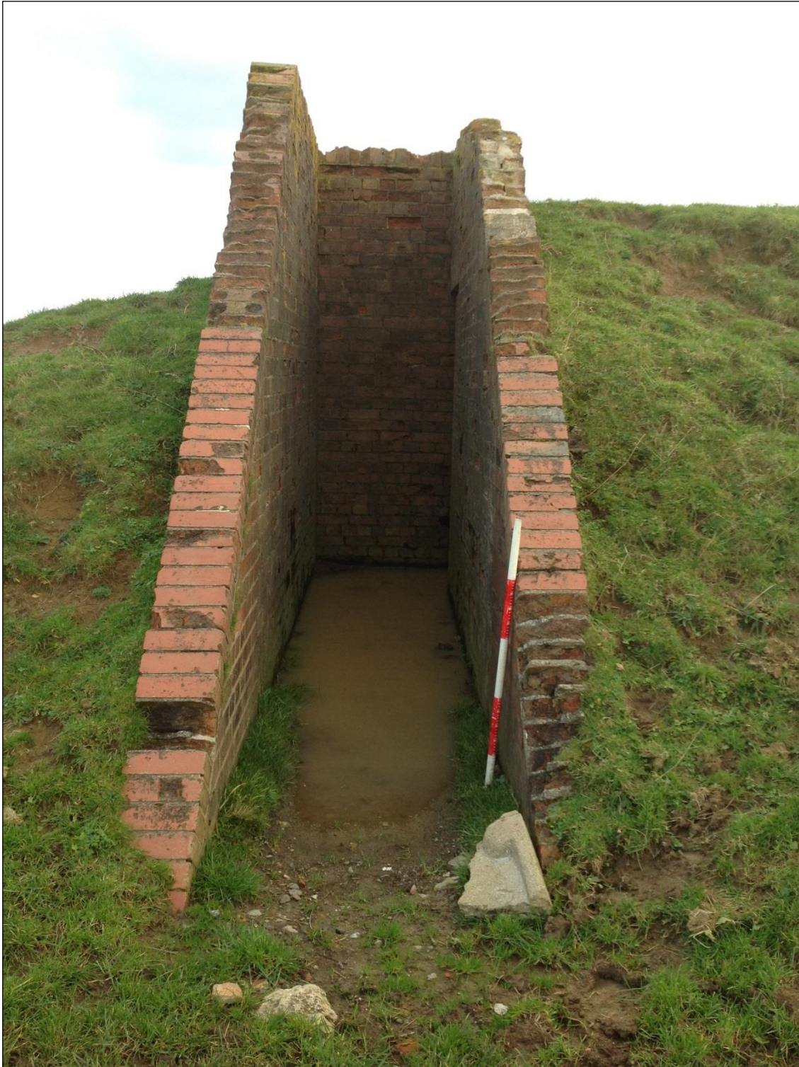
Plate 106: The brick blast walls protecting the air raid shelter entrance.
