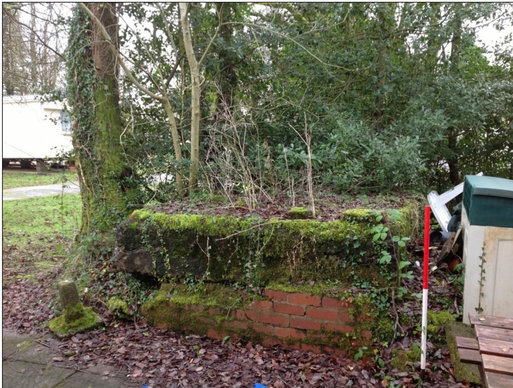
Plate 33: The reinforced plinth to house the site generator
