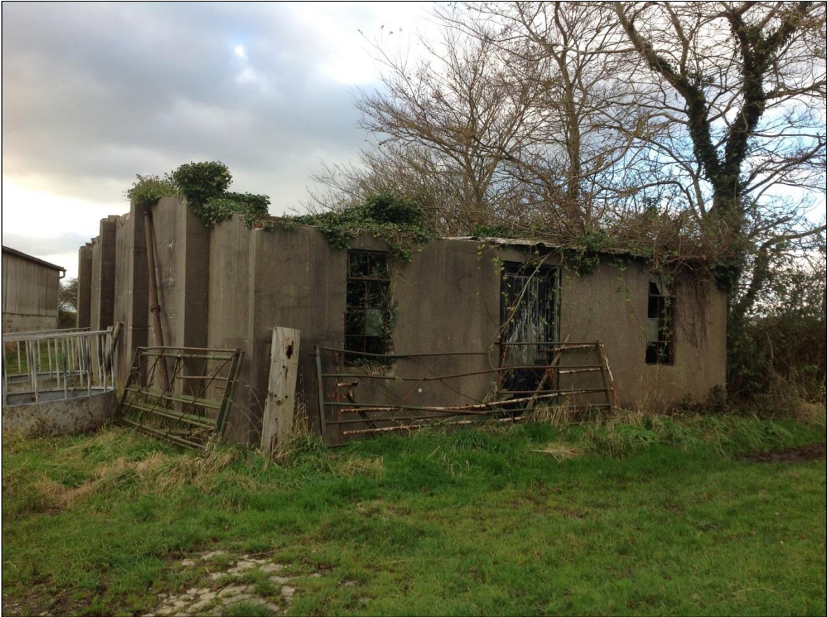
Plate 92: The heavily damaged remains of the Sites Squash Court. The main building should actually be double in height.
