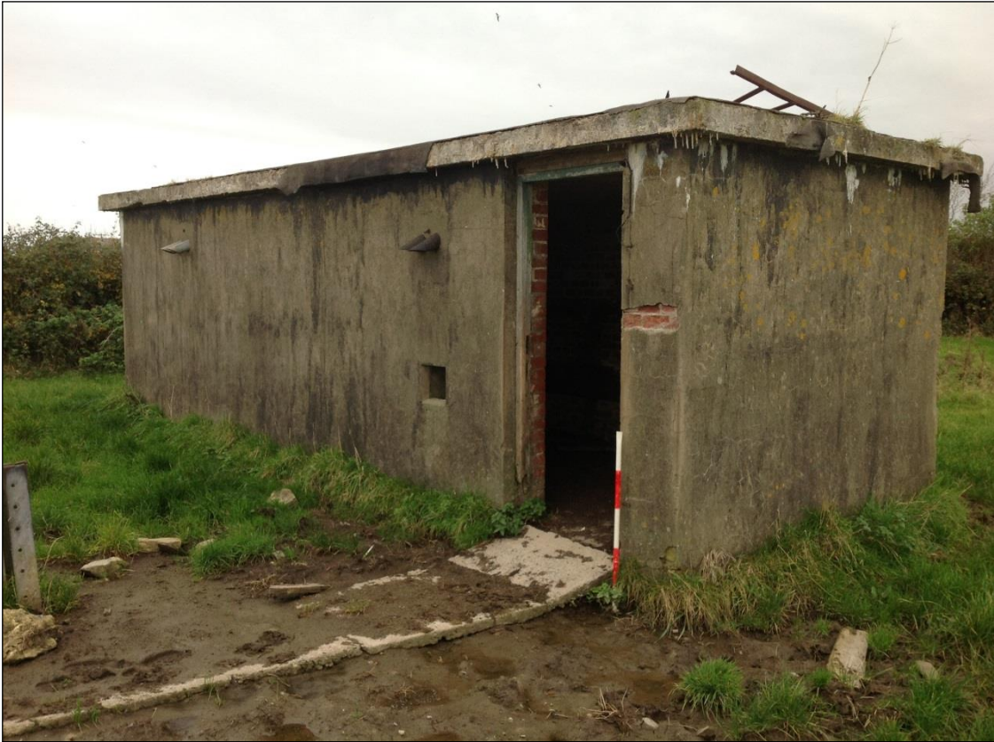
Plate 128: The VHF receiving station block. View to the northwest.
