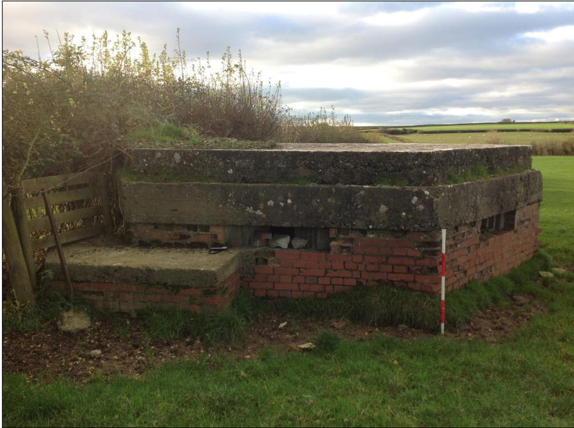
Plate 136: This pillbox, along with PRN 04470s, to the northwest, and 04185s, to the northeast, are of the same constructional type.
