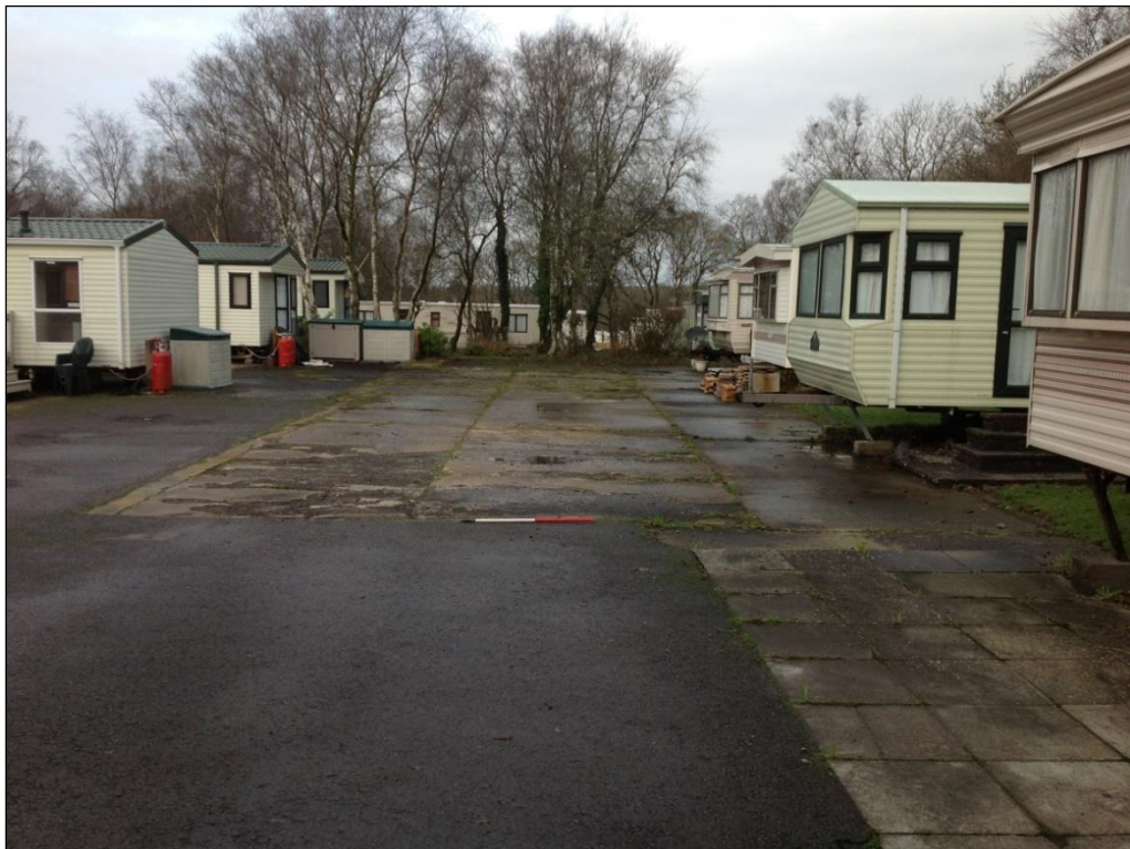
Plate 26: NAAFI Building (part of the Institute & NAAFI structure)
