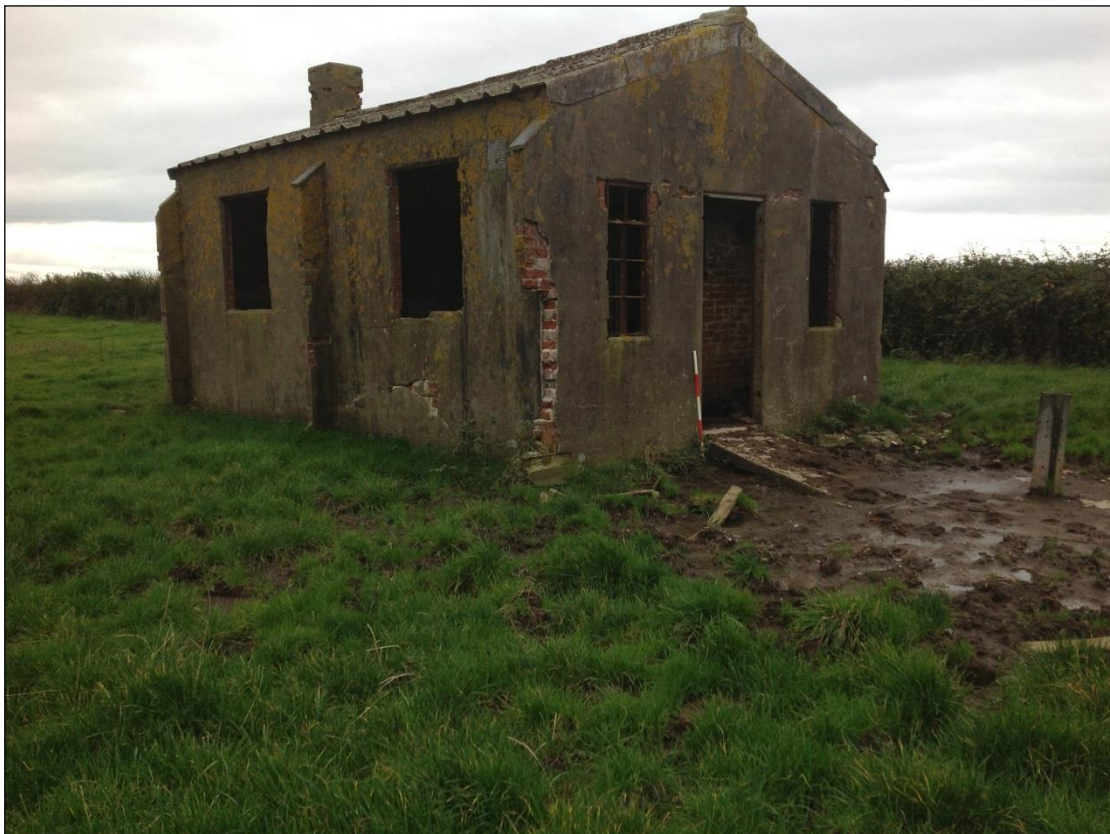
Plate 127: The VHF Rest hut. View to the south.
