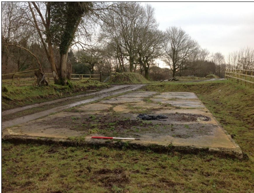
Plate 41: Concrete apron on which the Officers Quarters stood.
