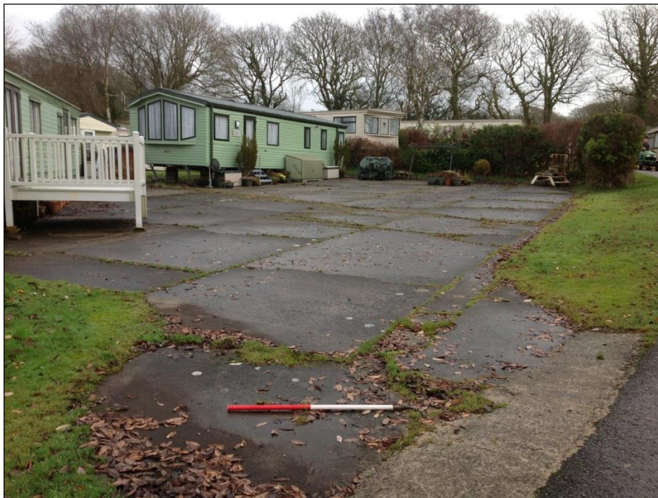
Plate 23: All that remains of the sites fuel compound.
