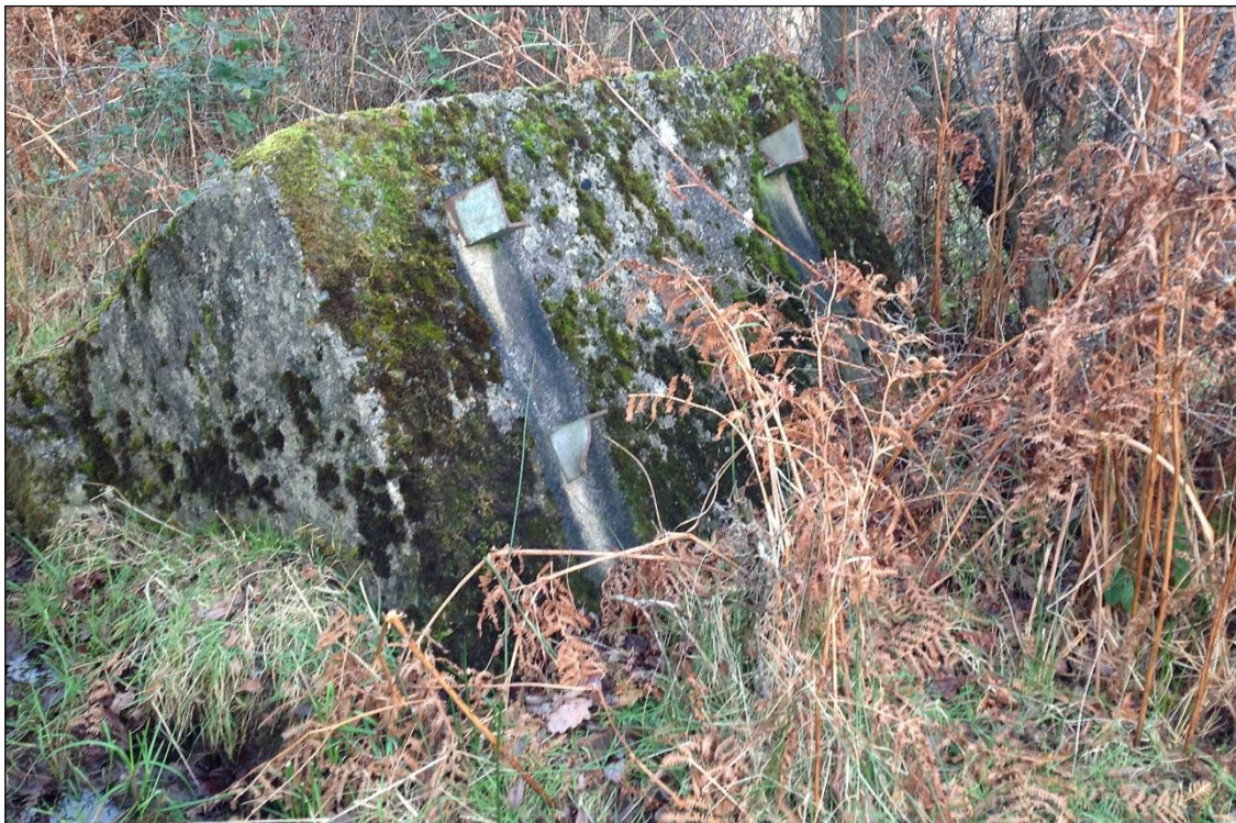
Plate 155: Concrete block of unknown use.
