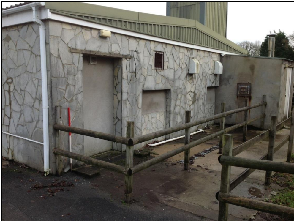
Plate 18: The front elevation of the decontamination annex. Note the sites of the projecting porches, the bin storage area between them and the site of the footbath tray which are all clearly visible.
