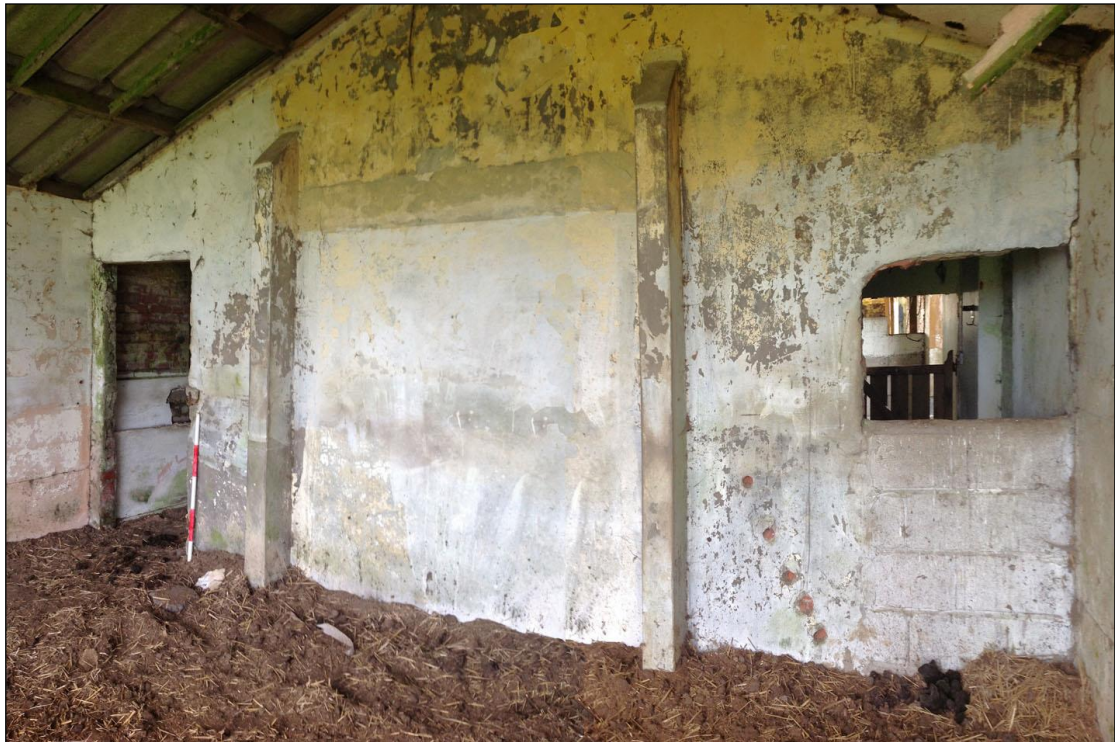
Plate 123: The interior of the Mess extension. Note the external piers on the interior wall. This wall would have been the original gable end of the building.
