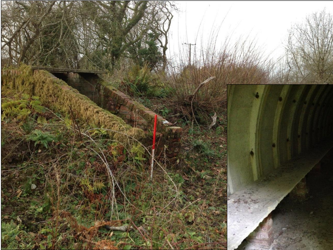
Plate 10: Air raid shelter. Concrete skimmed internal seating.
