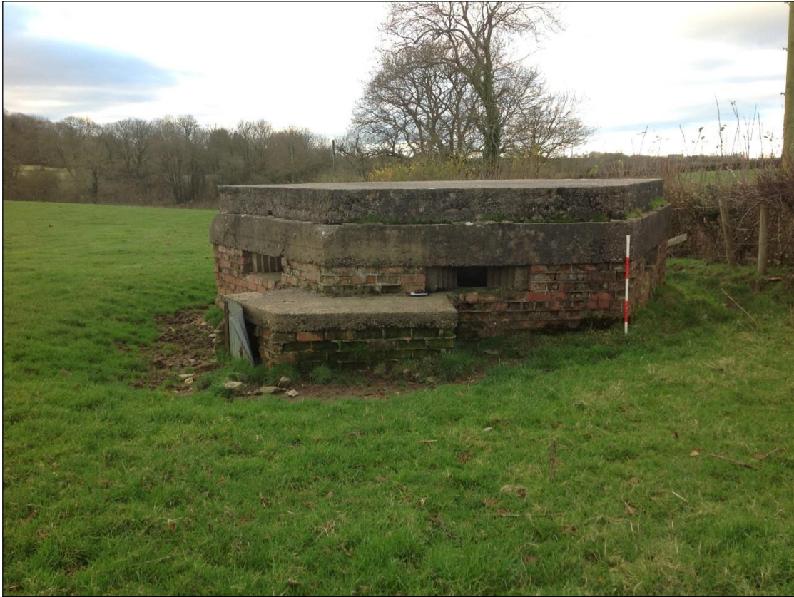
Plate 134: Pillbox PRN 04470s. View to the west.
