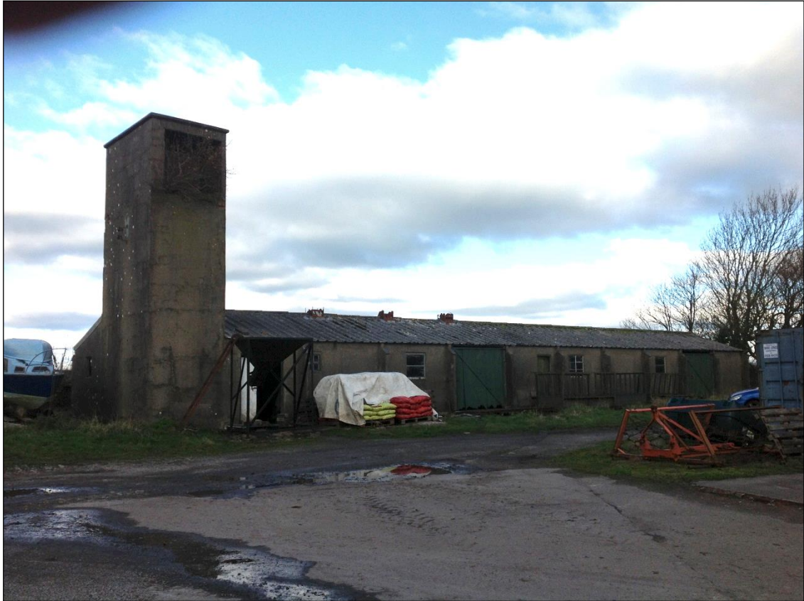
Plate 93: The Officers bath house. Note the removal of the external walls to make way for additional entrances.
