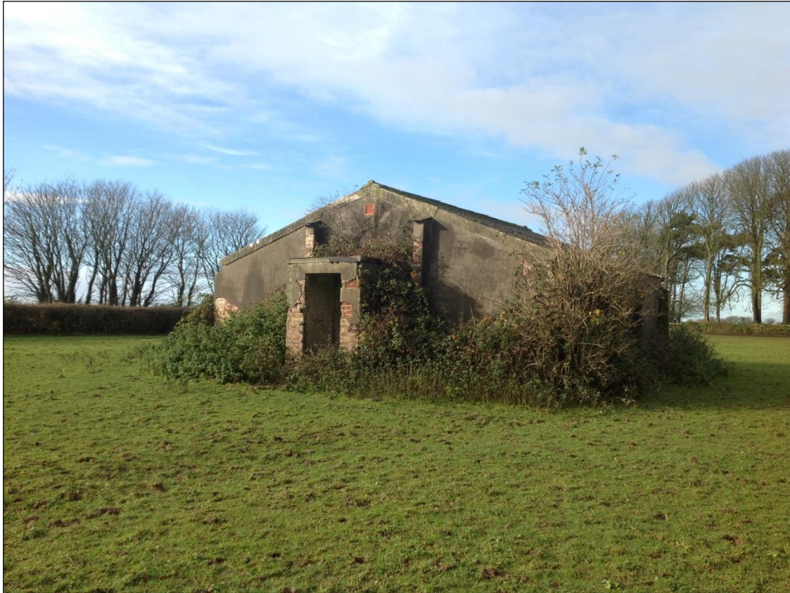
Plate 121: Southeast facing elevation of the recreation hut.
